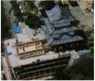
In 1995, Akashi Castle was seriously damaged by the Great Hanshin-Awaji Earthquake. Portions of the tower walls peeled off, and the stone walls collapsed in several places, including at the bases of the towers. In order to repair the stone walls under the towers, the towers themselves were raised on jacks and moved along a rail. This was the first time this technique of whole structure relocation was used in Japan.
